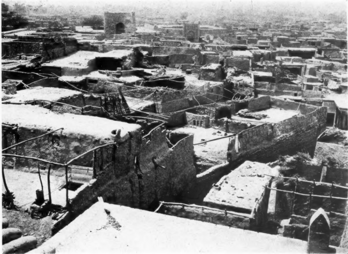
▲ THE CITIES are built of sundried brick over a structure of beams and sticks. A view looking over the housetops of Kashgar
